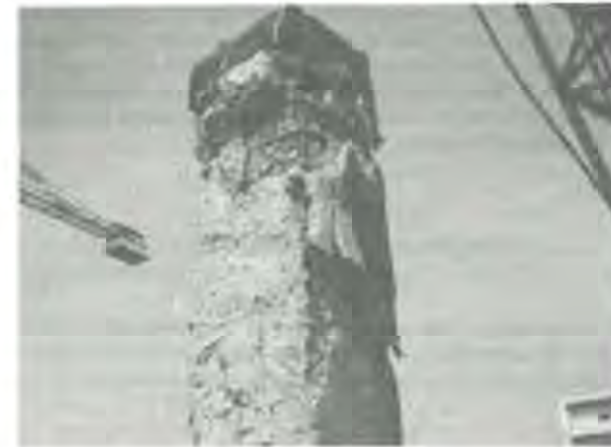
Figure 2. Example of brittle fracture of a pile made of concrete A.
