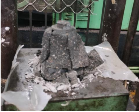
Figure 7: Typical concrete cone break out (SP6 G)
