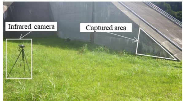
(a) Infrared thermography and captured area
