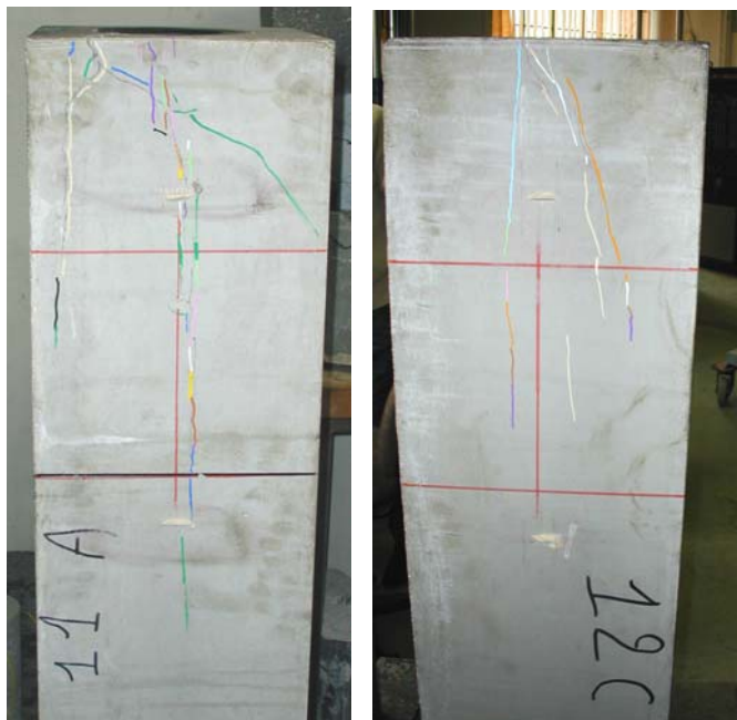
Figure 14. Progressive vertical development of splitting cracks (left) Block 11 side A, right) Block 12 side C.
