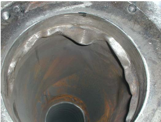
Figure 8. Local buckling of the duct at failure, block 7.
