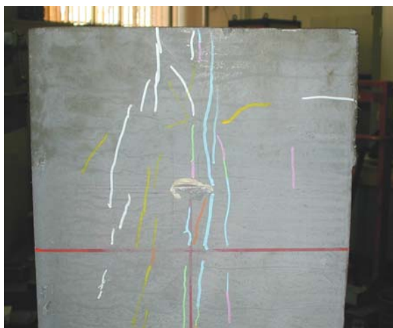
Figure 15. Progressive multiple cracking. Block 9 side C.
