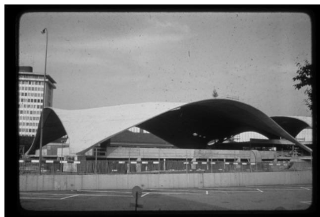
Figure 10. Sicli Building with no waterproofing.
