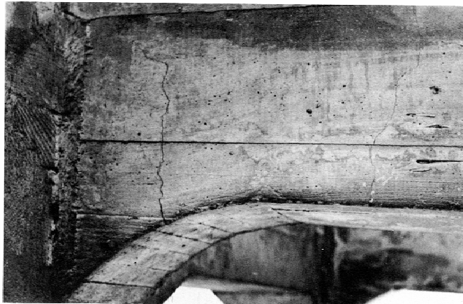
Figure 6. Aarburg Bridge and cracks.
