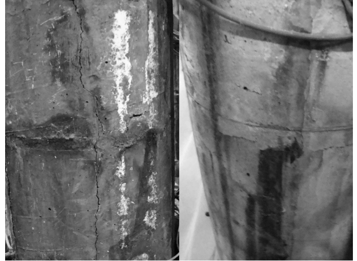
Figure 9. Cover surface cracking (longitudinal).
