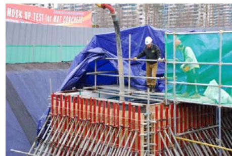
(b) Concrete placement
