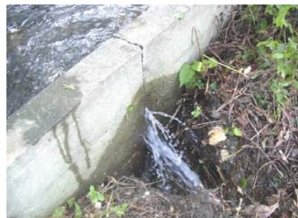
Figure 2. Water leakage from joint.
