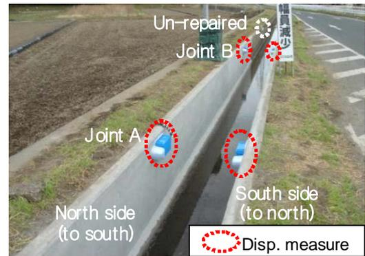
Figure 18. Completion of trial repair construction.
