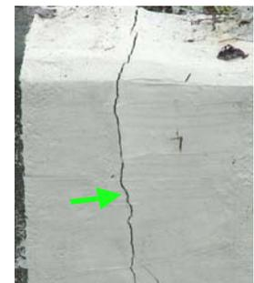
Figure 3. Crack generation in repaired part.
