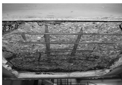
(b) Spray on mortar method
